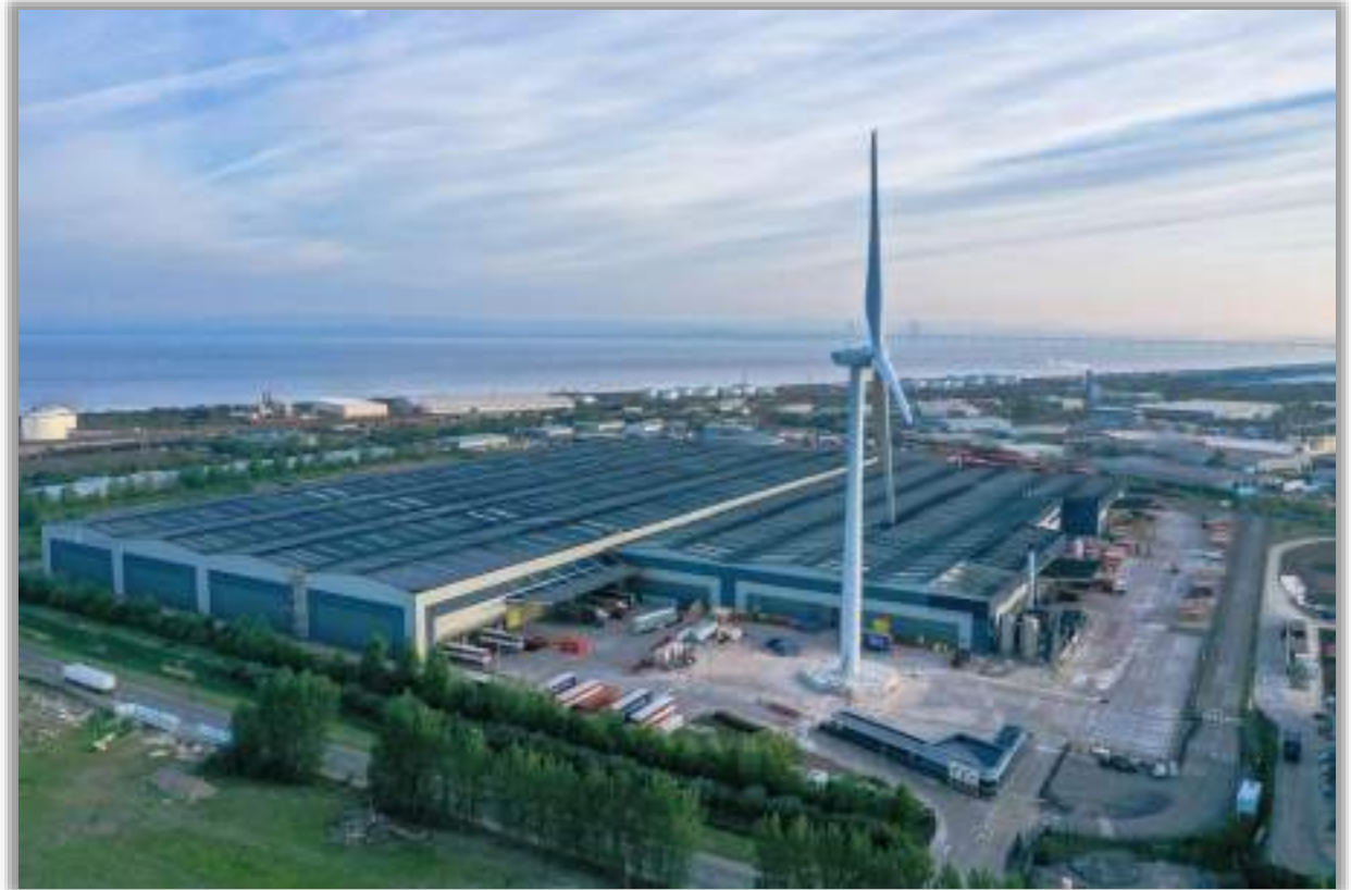
'The Park' beverages filling and logistics facilities in Bristol, England.
